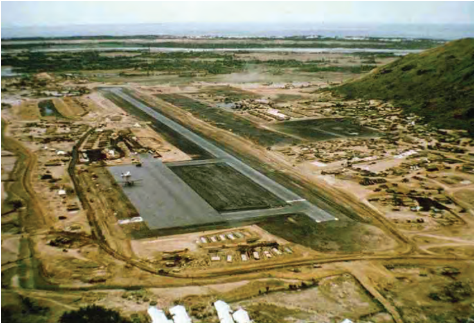
Once the airfield work at Duc Pho neared completion, the engineers turned their attention to reopening Highway 1 to Chu Lai.
